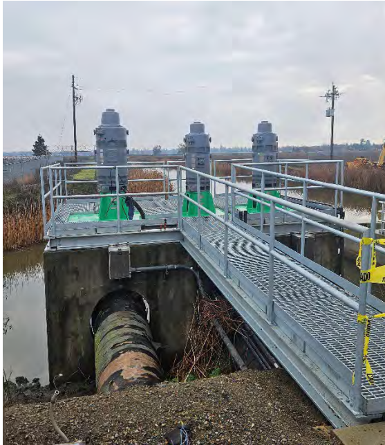
Rebuilt motors/pumps at Main Pump Station
