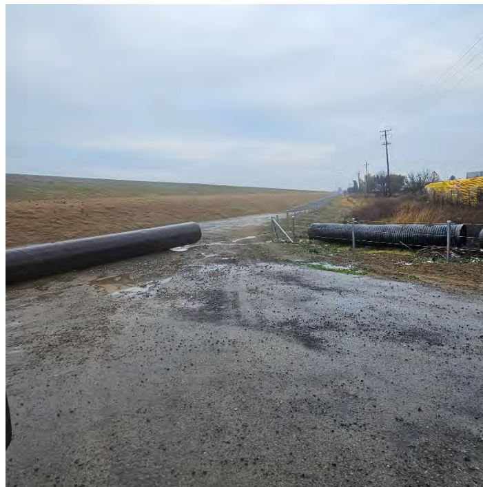
Yolo Bypass East Levee, South, completed berm
