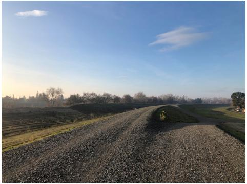
**Photo 3.** Photograph of the crown of the relocated Southport Levee, facing south. Notice the levee's original location to the east. The Project includes an ADA-accessible ramp that will provide access to the levee's crown (January 2021).
