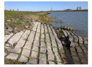
The two westernmost mats which are normally above the waterline are relatively undisturbed. The third mat near the waterline shows signs of disturbance, including the north edge which has rolled over, showing the rubber pads on the underside of the concrete blocks. The ropes securing the mats to the helical screw anchors and each other are under tension at the joint between the second and third mat.
